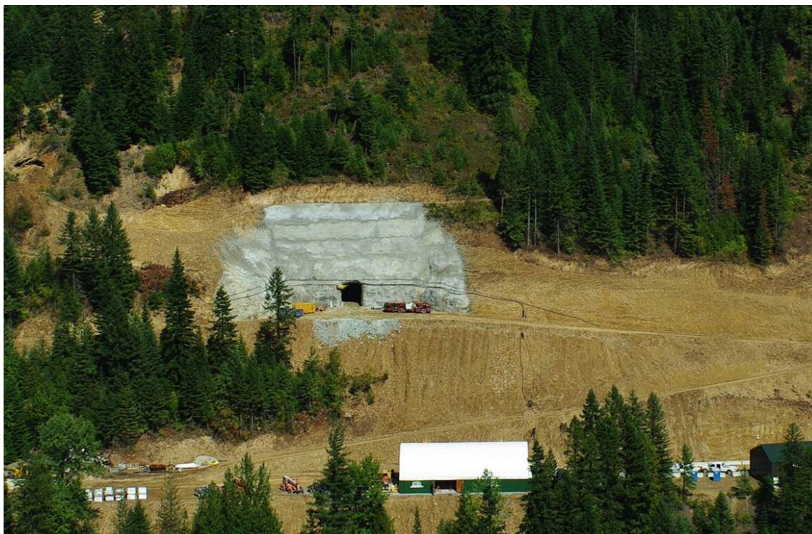
Figure 2 - Photo of New Golden Chest Mine Portal in October 2014
