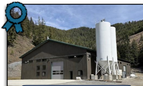
Murray Power Upgrade
